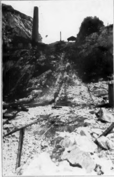
Incline from Bottom of Quarry.
